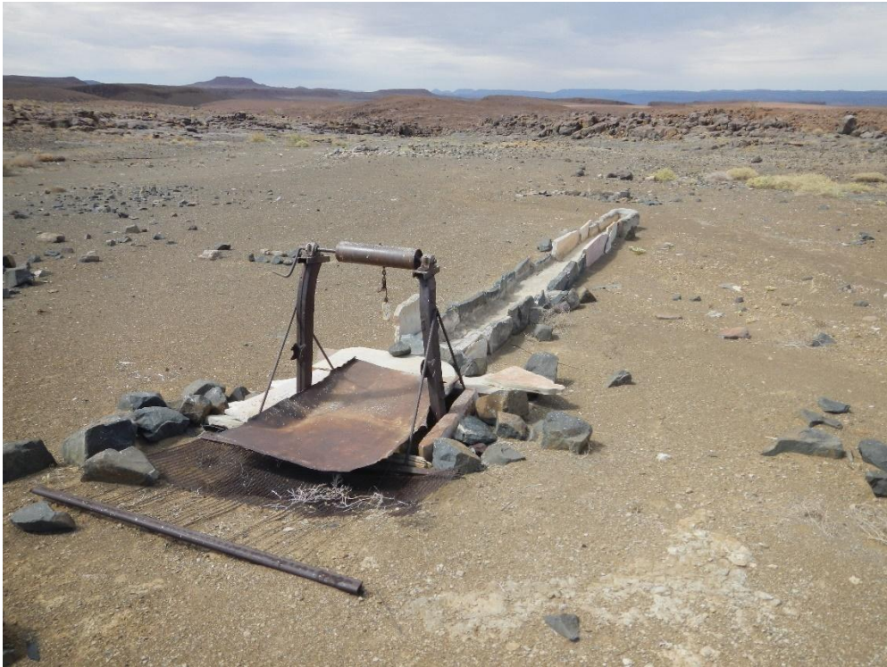
Figure 11: The well at Gams (QRS 10/44) viewed from the north showing windlass and stone watering crib. Note that the upright frame of the windlass is of relatively recent date having been made from the chassis of a Ford Model T and therefore post-dating 1908.
